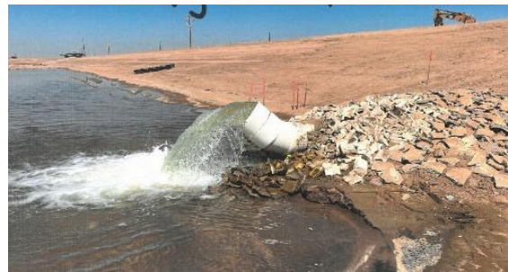
Figure 5 Pumping water from nearby canal to the infiltration basin.
